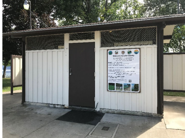
Third Street existing restroom
